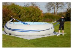
The belt must be positioned between the two loop supports. As you install the belt, secure it with the belt loops.
